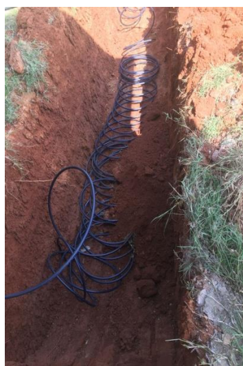
Figure 6.16 Air Conditioning by Geothermal Heat Pumps
