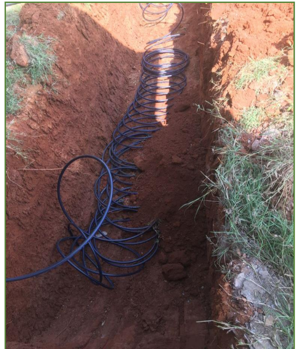
Figure 5.11 Model of air conditioning by geothermal heat pump
