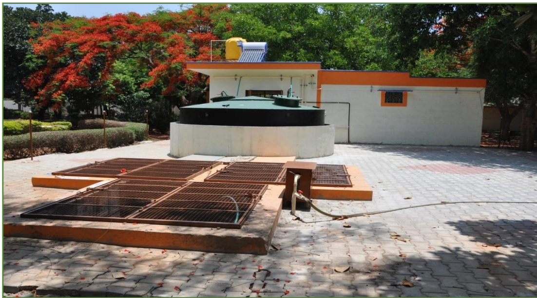
Figure 5.13 0.5 MT / Day – 500 Kgs per day capacity - Bio gas plant (SJCIT Boys Hostel)
