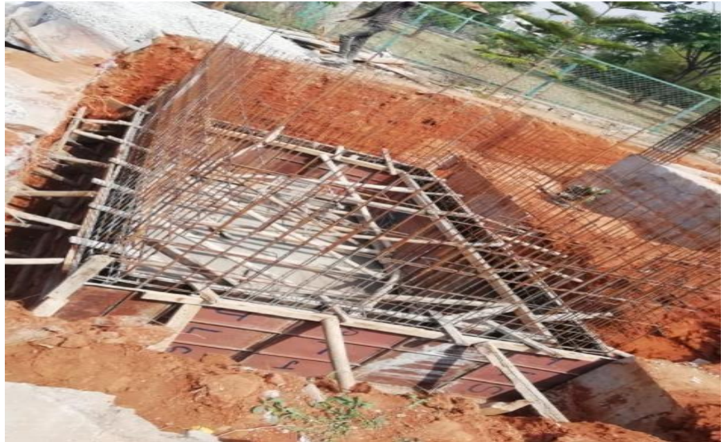
FIG. 7.6 SHUTTERING FOR CONCRETE FILLING
