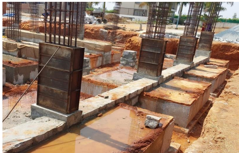
FIG 3.1 COMBINED FOOTING AND INDIVIDUAL FOOTING
