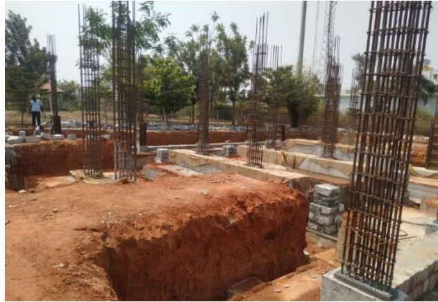
FIG 4.2 COLUMN STARTER
