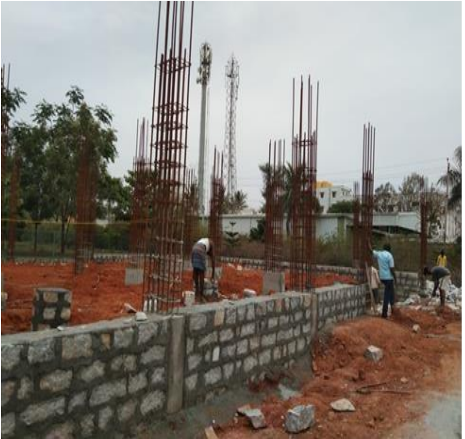
FIG 5.1 SIZE STONE MASONRY
