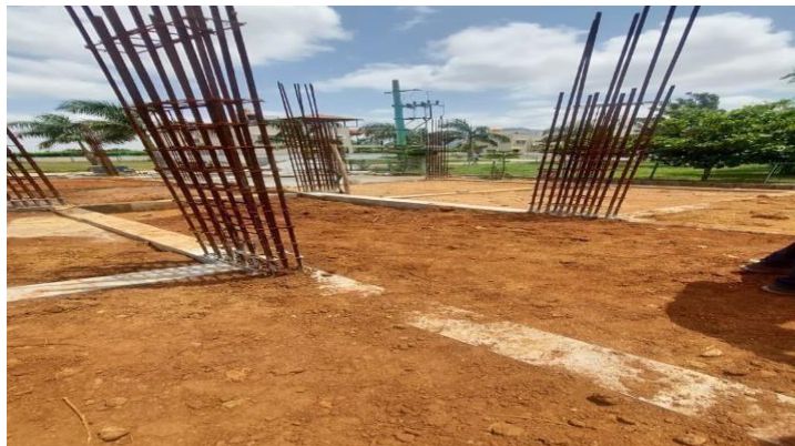
FIG 6.7 FILLING IN FLOORING
