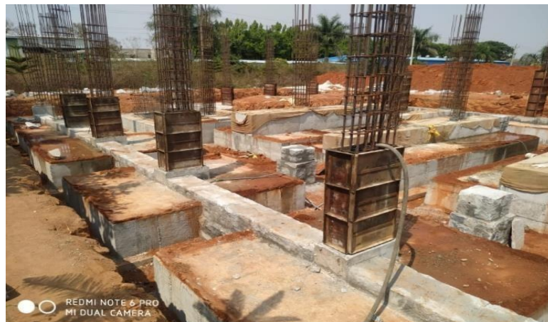
FIG 4.3 COLUMN SHUTTERING
