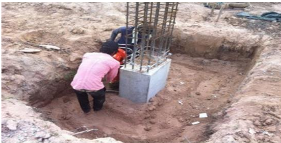
FIG 6.2 FILLING IN FOUNDATION.
