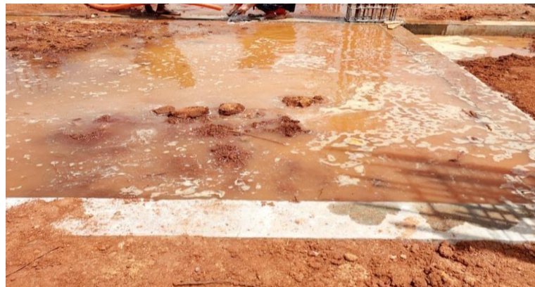
FIG 6.8 CONSOLIDATION AFTER FILLING
