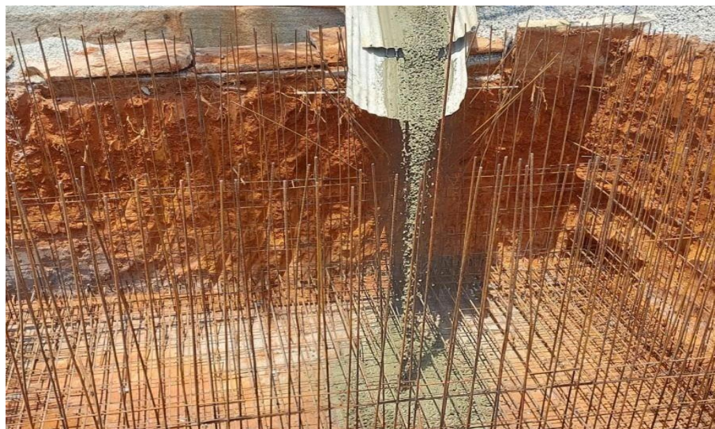
FIG 7.5 SLAB CONCRETING
