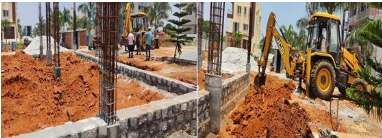
FIG 6.1 SAND OR EARTH USED IN FILLING WORKS
