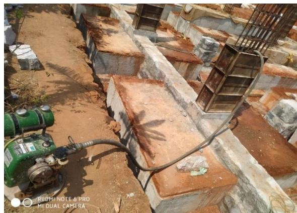
FIG 4.4 COMPACTION BY MECHANICAL VIBRATOR
