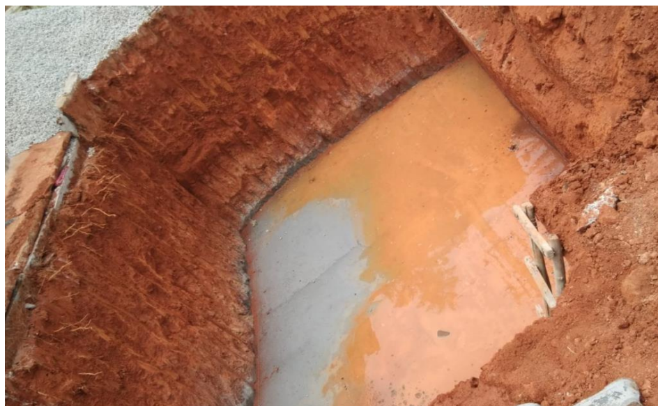
FIG 7.3 PCC BED CURING
