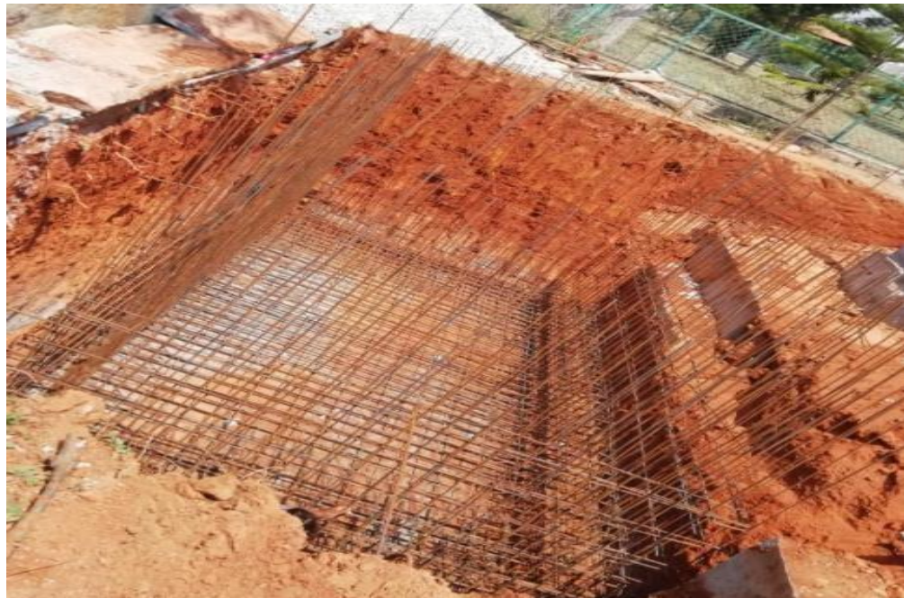
FIG 7.4 REINFORCEMENT OF WATER TANK
