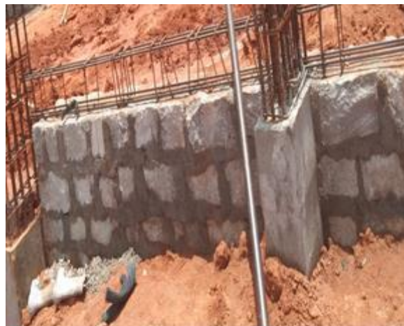
FIG 6.5 STEEL BARS IN PLINTH BEAM
