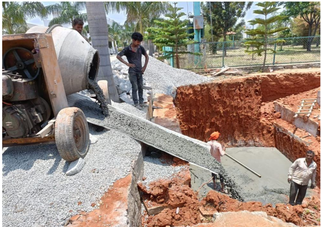
FIG 7.2 PCC BED FILLING
