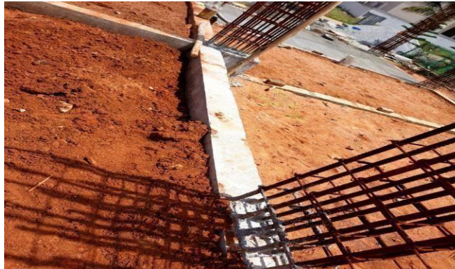
FIG 6.6 FILLING IN PLINTH BEAM
