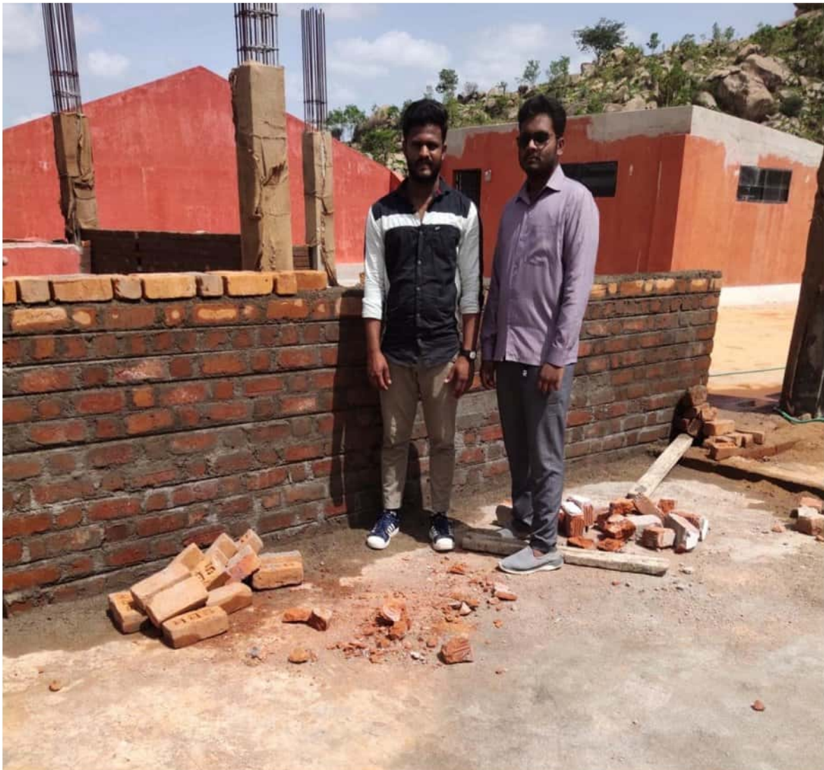
Fig:4.6 CONSTRUCTION OF BRICK WALL
