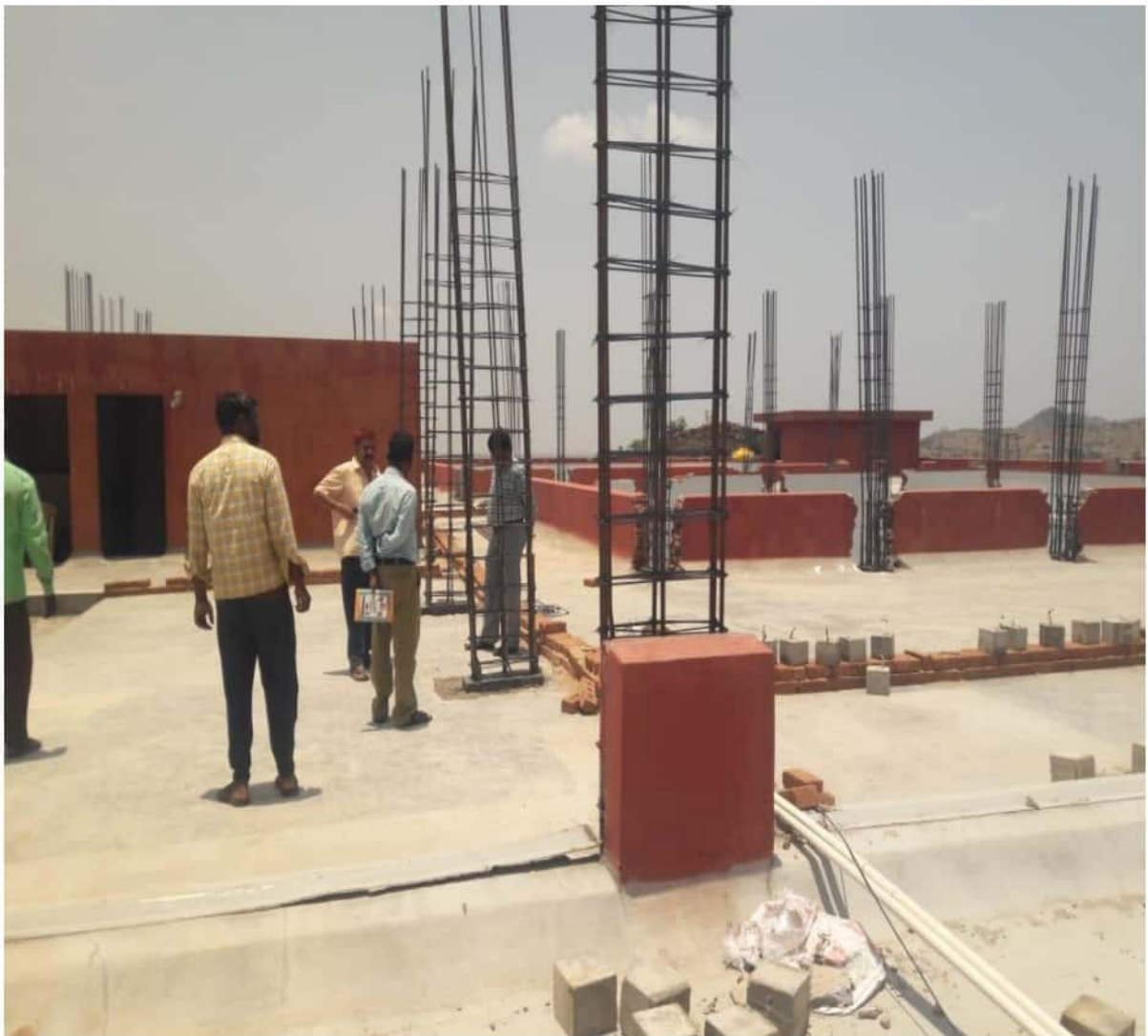
Fig:3.6 COLUMN REINFORCEMENT
