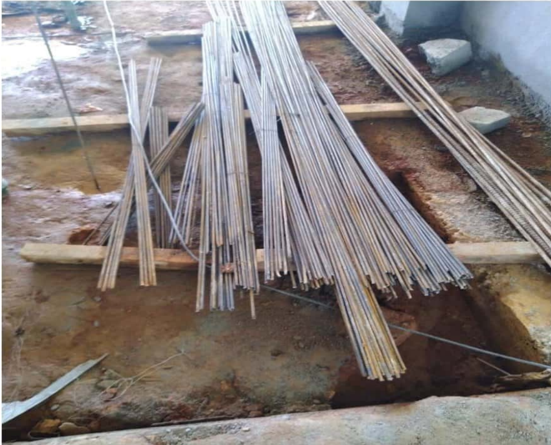
Fig$:3.4 REINFORCEMENT BARS
