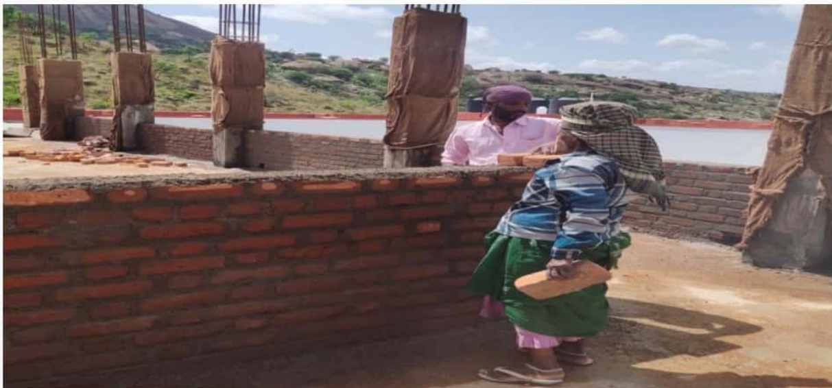
Fig:4.5 CONSTRUCTION OF BURNT BRICK MASONRY WALL
