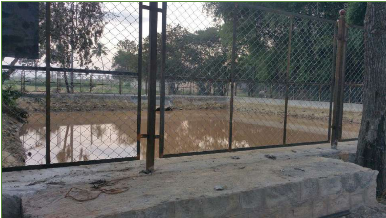
Figure 5.17 Water Pond of 35 lakhs liters capacity
