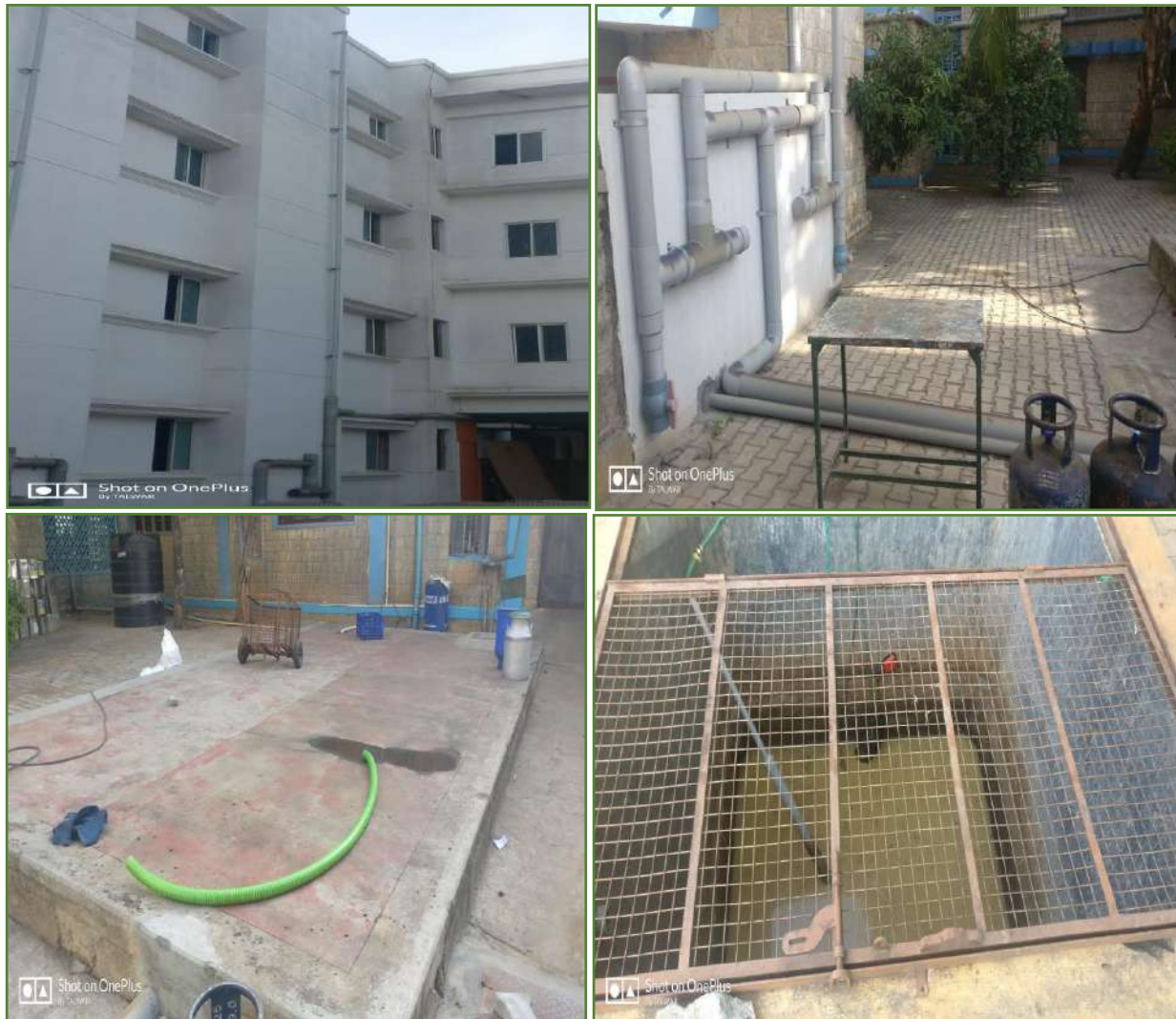
Figure 5.16 Rain water harvesting for SJCIT boys hostel
